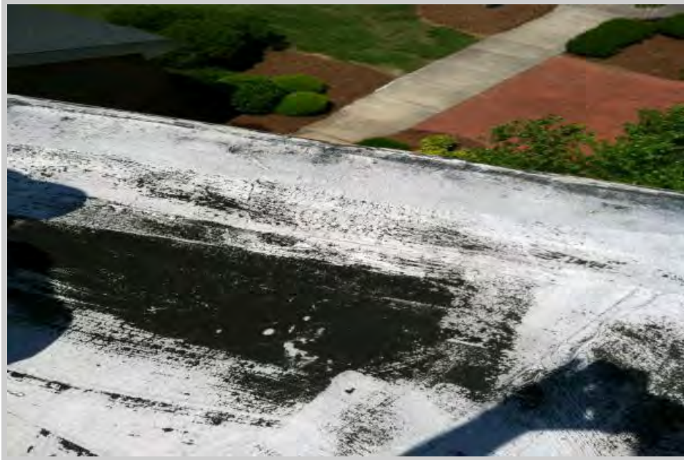
The top membrane ply has separated from the perimeter metal edge.
