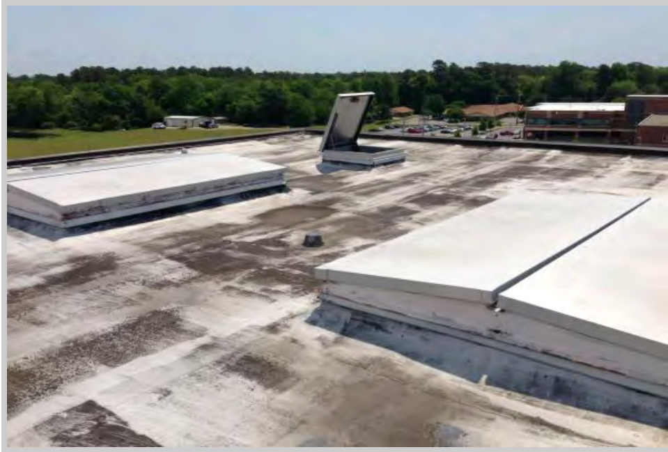
The rooftop penetration flashings are in fair shape. The trapped moisture is running from the building perimeter.
