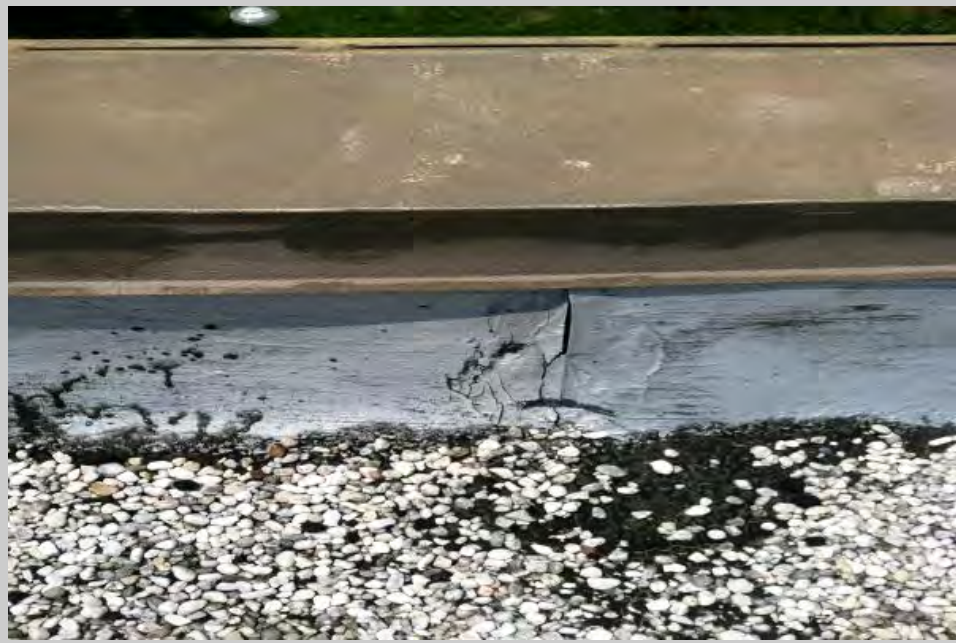
Rooftop view of open lap joint on the base flashing.
