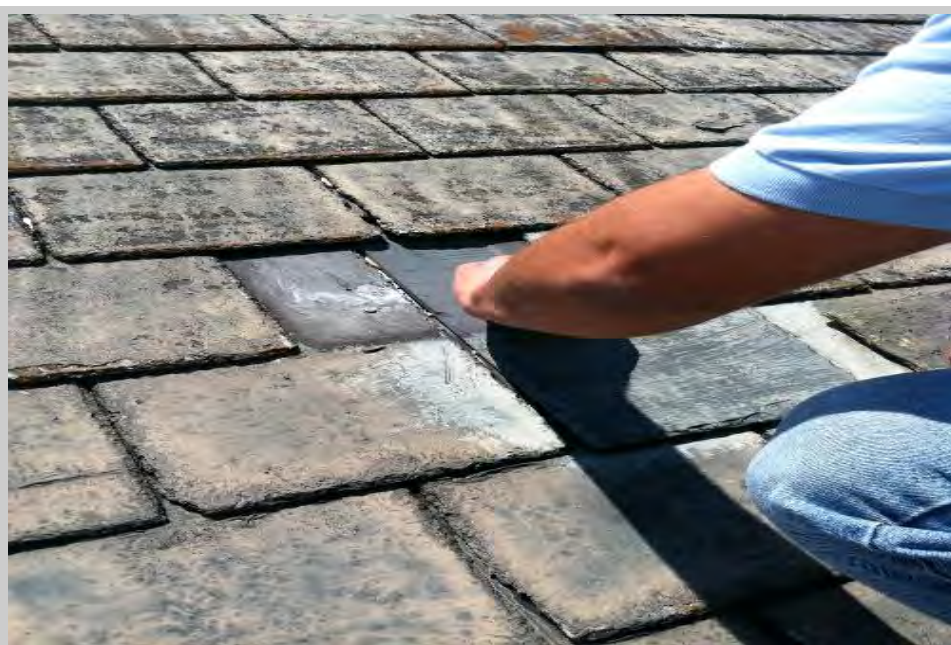
Rooftop view of the condition of the asbestos shingles on the building C. The College of the Albemarle Maintenance department has been very proactive and reactive in replacing worn or blown off shingles over the years.
