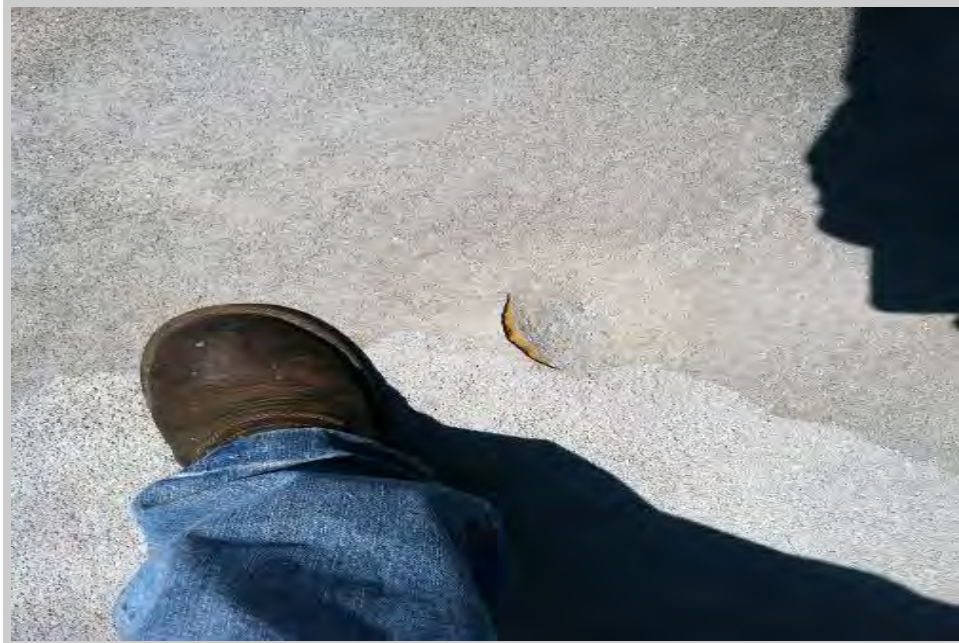
Asplit in the sprayed polyurethane roof section.
