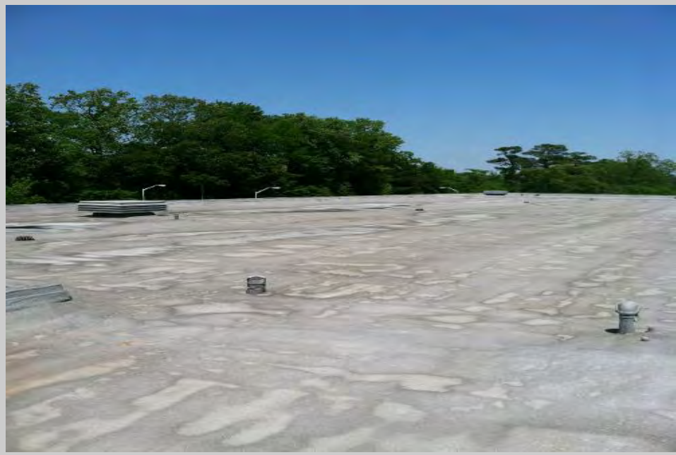
Roof Overview of the sprayed foam polyurethane roof system coating.
