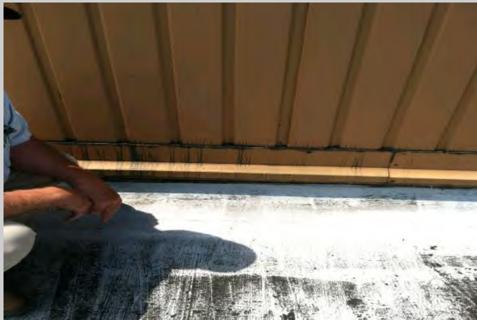
Most of the reported leaks have been evidenced at the roof/wall panel transition as well as the perimeter edge metal detail.
