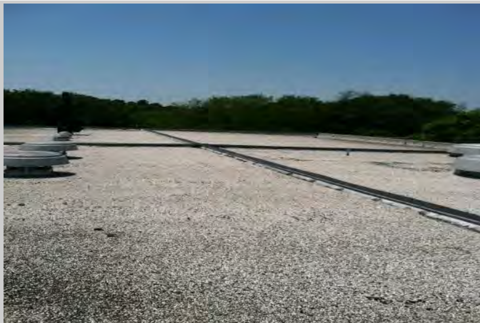
Rooftop view of aged expand o flash neoprene expansion joint. Some preventative maintenance has been performed on these suspect roof transition points.
