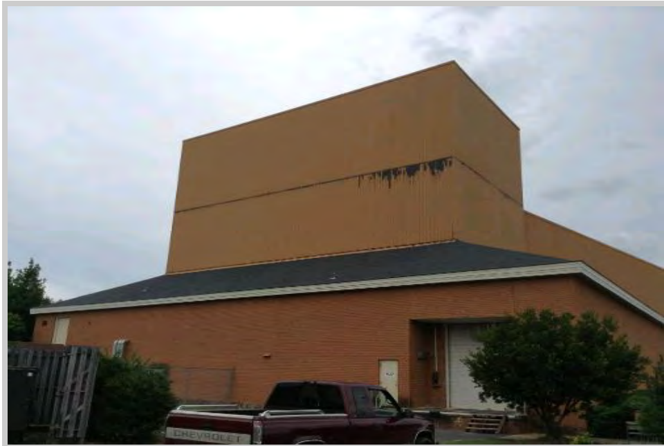
Front view showing oxidation and chipping paint on the upper auditorium wall panel system
