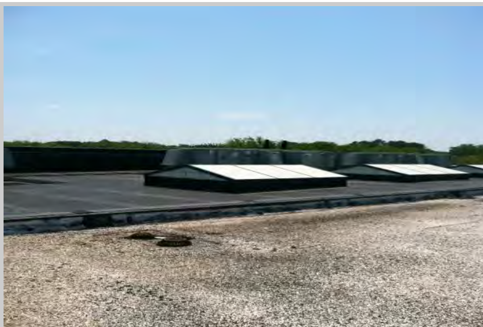
Rooftop view of aged low base flashing.
