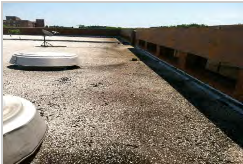
Wall flashing that needs to be stripped in with a new base and cap sheet.
