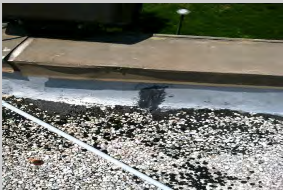
A rooftop view of a loose metal coping cap and repaired base flashing detail.
