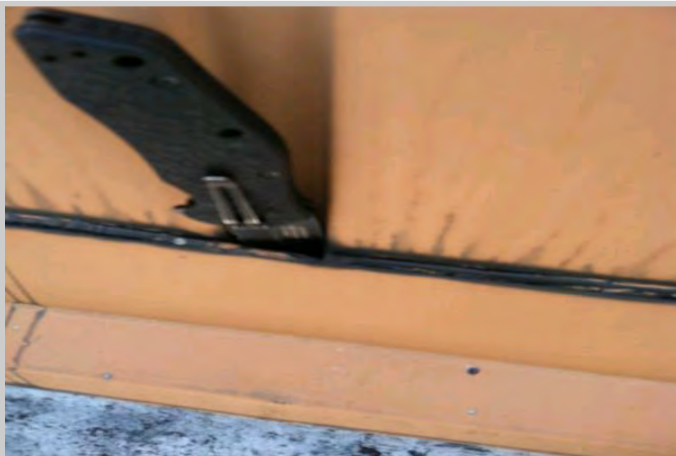
A close-up view of the deteriorated sealant detail at the wall panel roof flashing transition.
