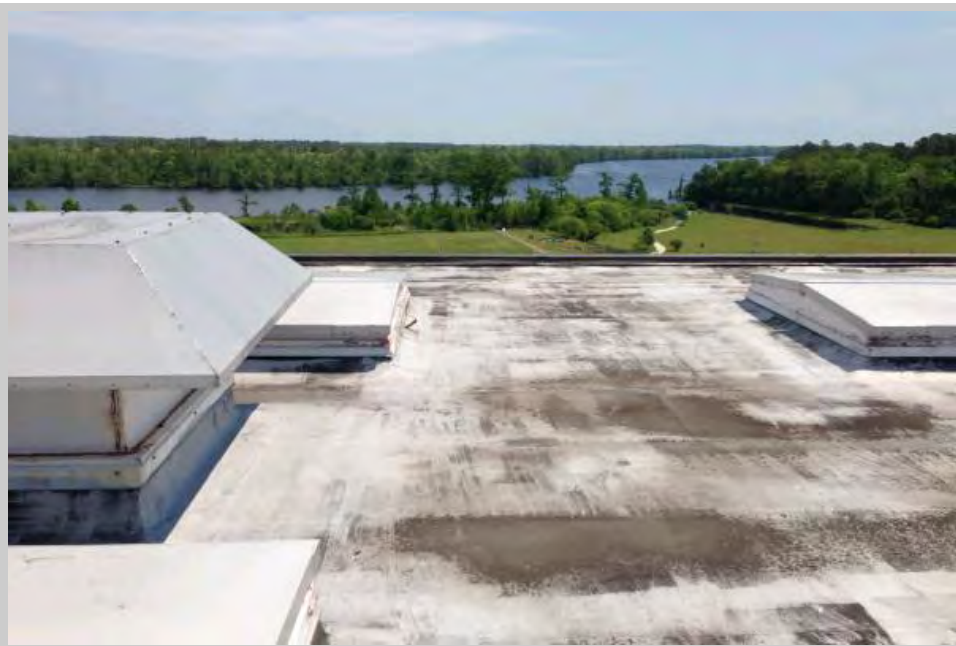
The perimeter edge metal has failed allowing moisture to migrate to the field of the roof.
