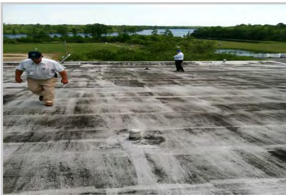
Rooftop view of the built-up roof system. Note the nice slope but the degrading roof coating protection layer.
