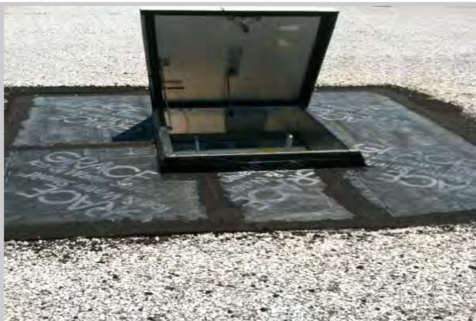
The College of the Albermarle maintenance dept has installed a temporary solution peal and stick membrane slowing the water flow into the building envelope around this roof hatch.
