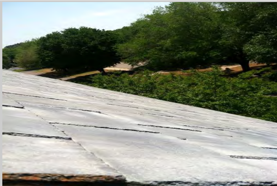
Rooftop view of the Library mansard asbestos shingles. Note the great slope that has prolonged the life of the shingle. Many shingles are loose or have been repaired/replaced.
