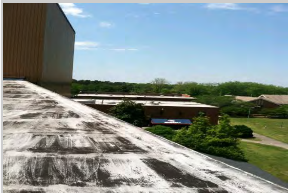
The entire perimeter edge detail needs to be stripped in additional roof plies. Evidence of moisture migration noted at several open points in membrane laps.
